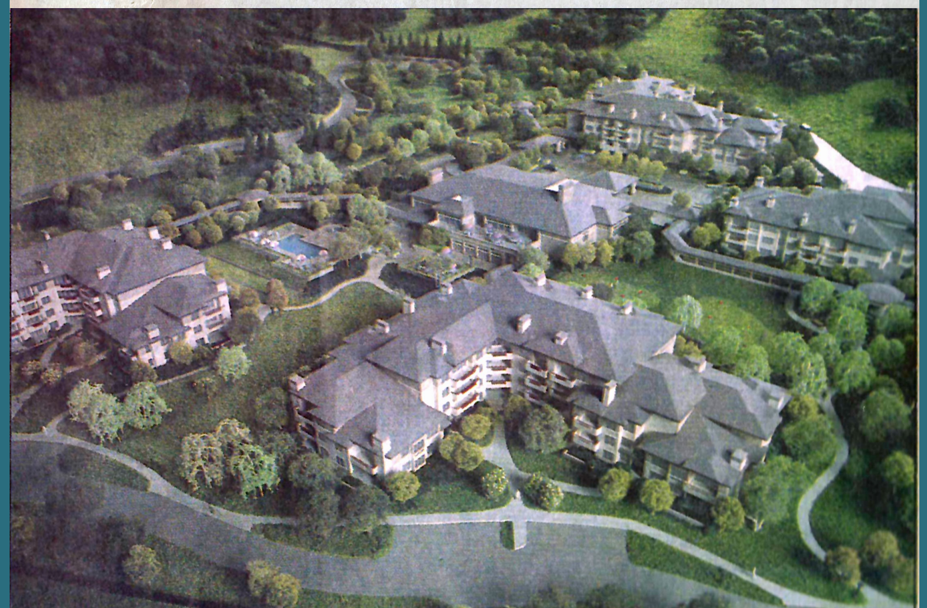
Smith Ranch Homes was to be built at the level of the very best condominiums with the qualities needed to satisfy a group of successful people who are living well.
